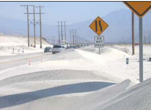
Windblown sand hazard along Indian Canyon Drive.
