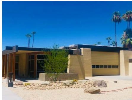
Fire Station No. 4 on Laverne Way in South Palm Springs
