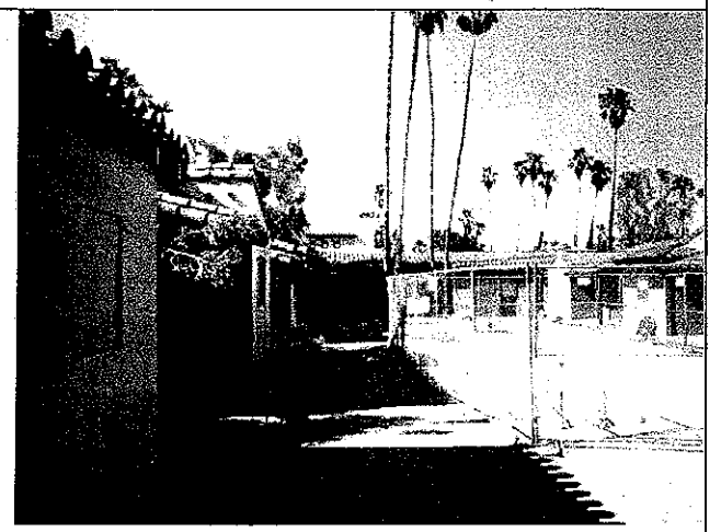
Bungalow sidewalk (Label C)
