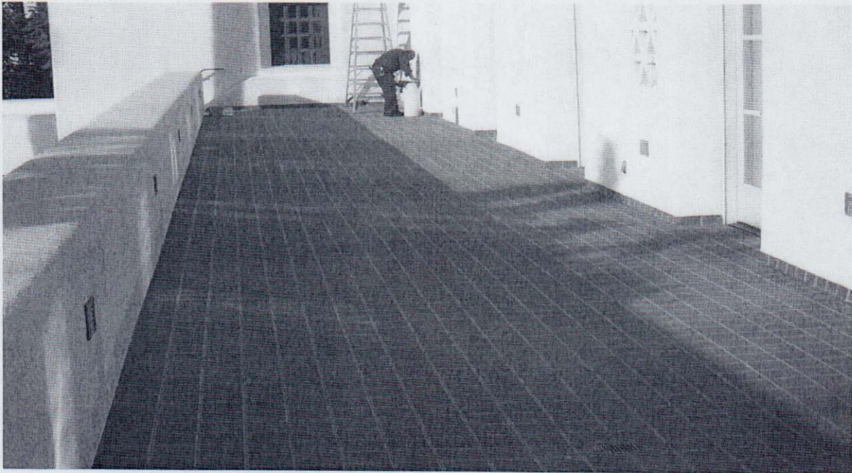
Existing balcony colored concrete deck to be removed
