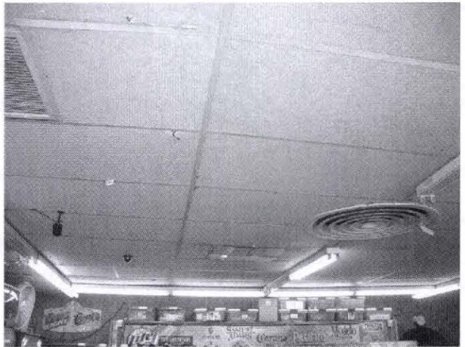
Retail Space Ceiling
