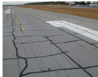
Block Cracking
