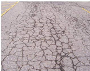
Alligator Cracking
